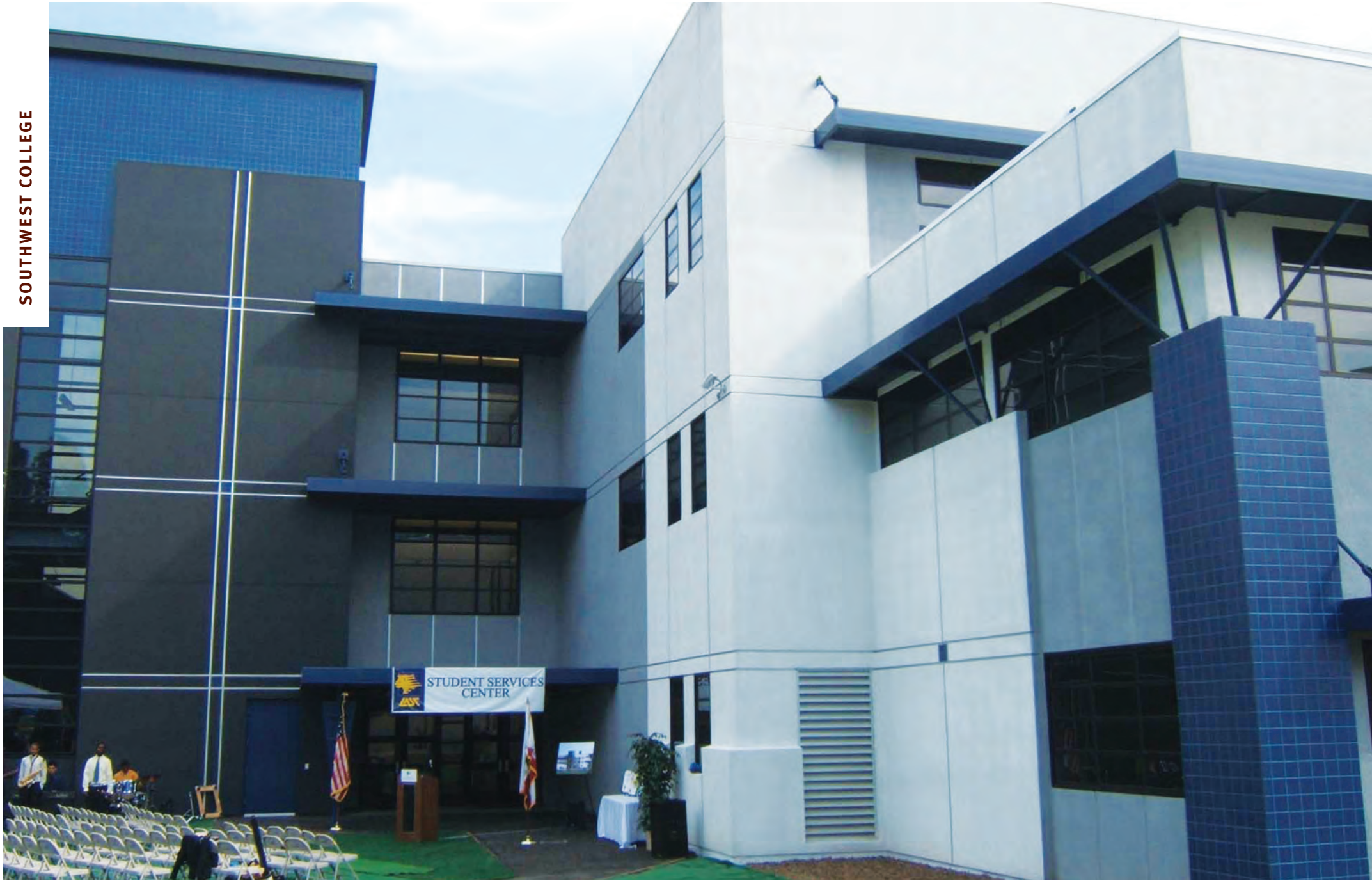
Last year, Southwest College celebrated the opening of the new Student Services Center. The 62,000 square foot building helps the College better serve the LASC student population by centralizing student services under one roof.
